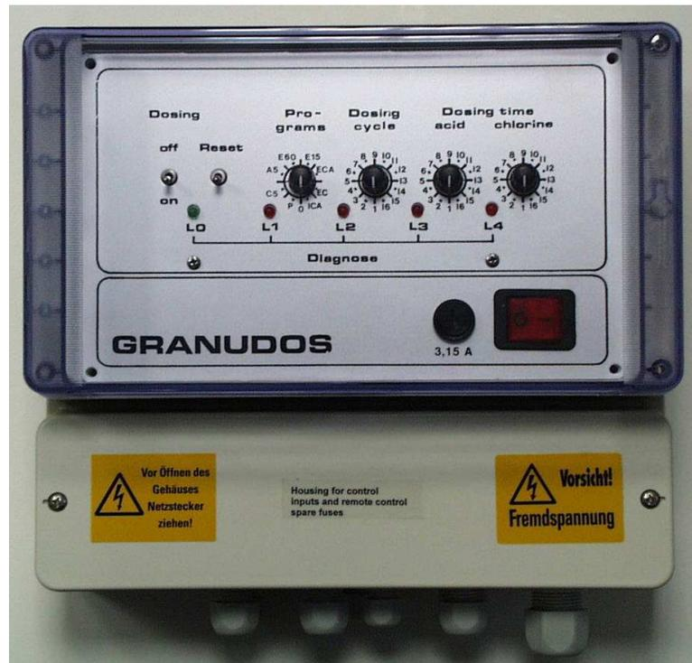
The control system is enclosed within a dust proof and splash proof housing (IP 65). External switches and fault remote indication are to be connected in the lower part of the housing.
